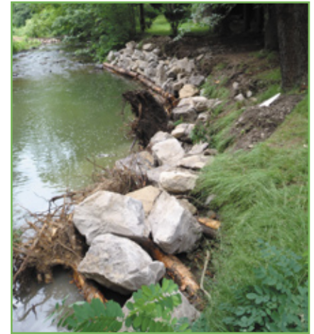
After: the same bank with boulders, log cribbing and root wads installed.
