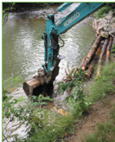
Positioning bank cribbing logs
