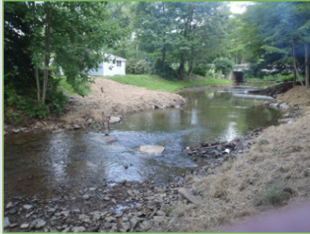
Upstream view of finished log vanes
