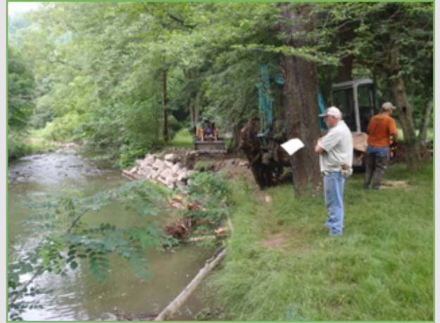
Another view of bank cribbing construction
