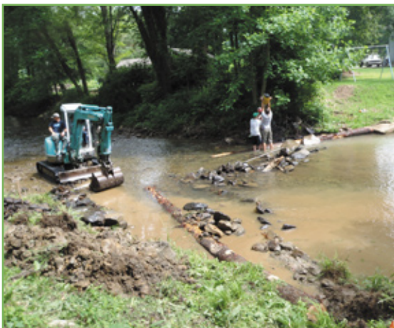
Constructing log vanes that will create a deep run
