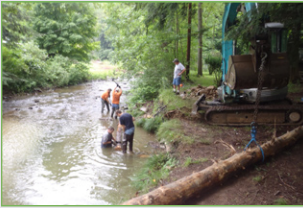
Construction of bank cribbing
